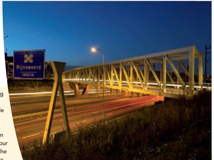
Figure 1 - The A27 bridge, the longest hybrid composite bridge in the world. ©DSM
