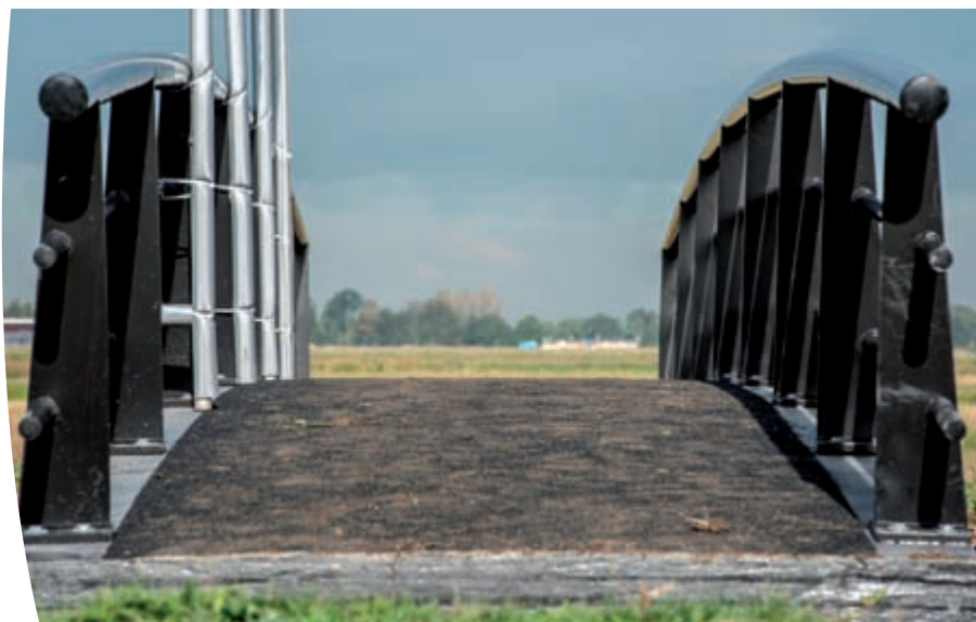
Figure 2 - First bridge made from bio-based raw materials. ©DSM
